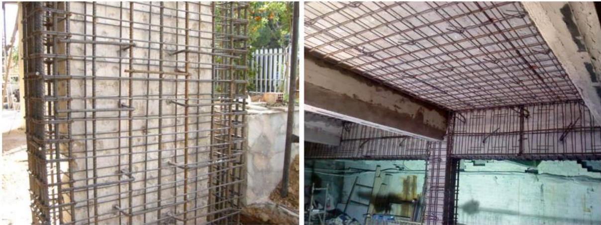
Figure 3. Seismic upgrading with RC jacketing
