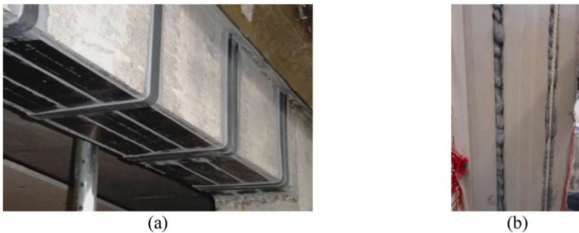
Figure 7. (a) Flexural and shear strengthening with FRP laminates; (b) flexural strengthening with NSM reinforcement [Source: Lecture notes, T. Triantafillou].
