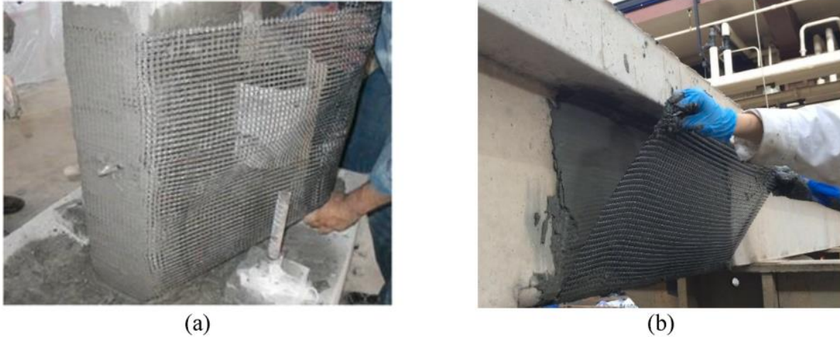
Figure 9. Applications of TRM jacketing on RC (a) column and (b) beam
