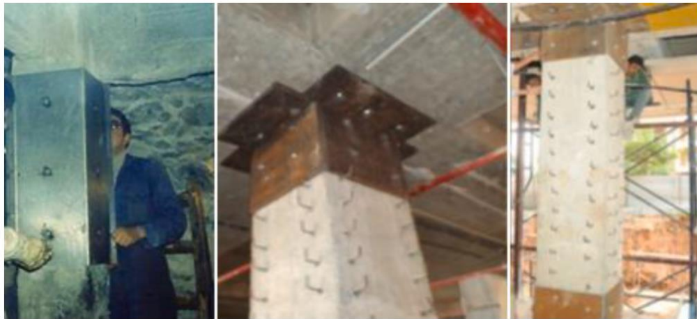
Figure 4. Seismic upgrading with steel jacketing
